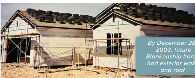
Framing in place
