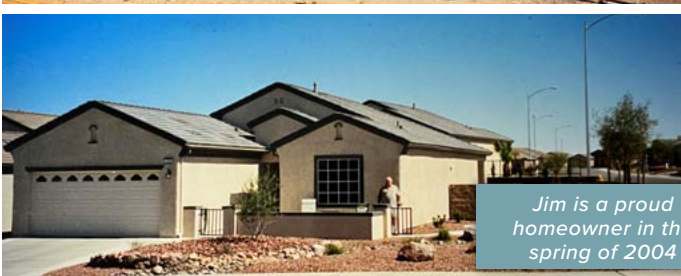
By December 28, 2003, future Blankenship home had exterior walls and roof
